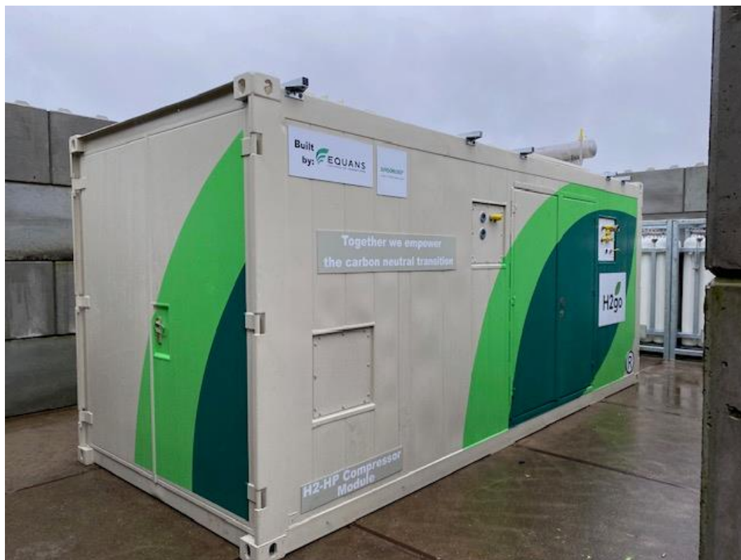
Compressor module Smart Energy Hub Hessenpoort Zwolle ( www.h2-go.nl )
